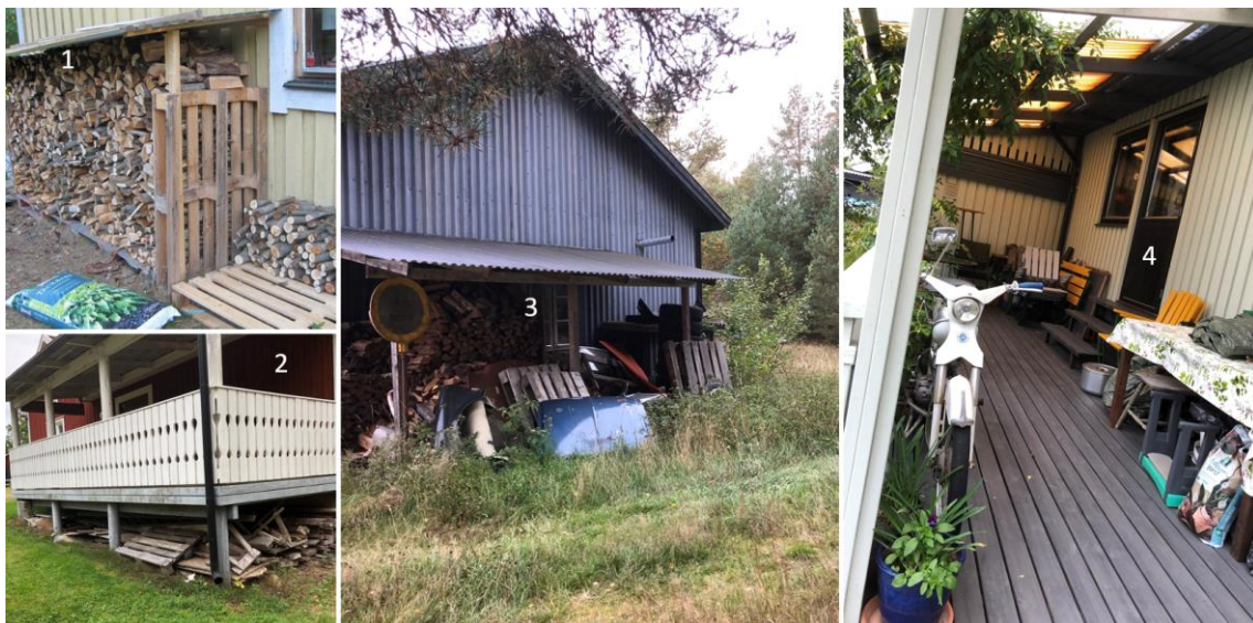
Figure 31. Non-vegetation fuels in semiconfined spaces directly adjoining homes. (1) Characteristic wood fuel pile with metal rain protection in suburban townhouse. Photo: Stella Norrvi, with permission. (2) Wooden porch with wooden roof and timber storage under the floor in rural dwelling. (3) Storage of wood fuel, car tires, wooden pallets and miscellaneous under a metal rain protection at the façade of an industrial/storage outbuilding. The surrounding vegetation is unmanaged grassland. (4) wooden porch with plastic ceiling filled with combustibles, including an old motorbike.
