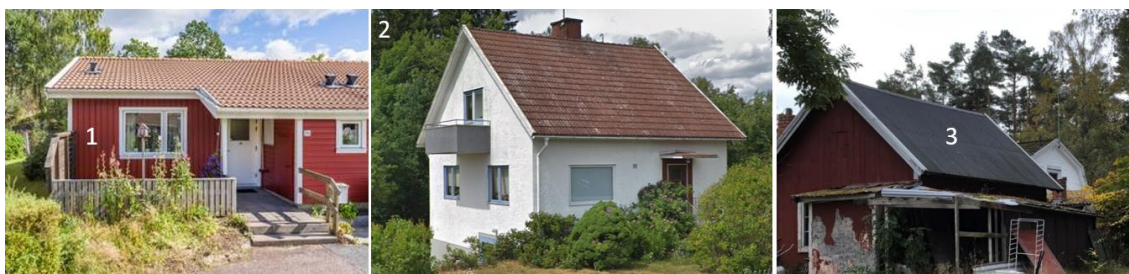
Figure 7. (1) Townhouse with timber façade and tile roof. (2) single dwelling with plaster (mortar) façade and tile roof. (3) Outbuilding with timber façade and metal roof.
